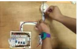
• Fit the ground cable (green cable) at the ground terminal. Then insert the ground cable from the distribution box to the round PVC block.
