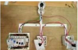
Screw the lamp holder and the switches. Then install the casing cover and the distribution board cover.
