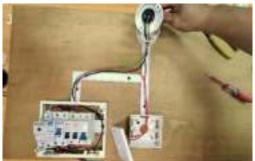
Screw the lamp holder and the switch. Then install the casing cover and the distribution board cover.
