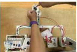
• Screw the lamp holder and the switch. Then install the casing cover and the distribution board cover.
