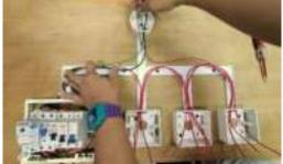
Fit the live cables at the first terminal box to the first two-way switch. The live cable
