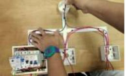
Fit the ground cable (green cable) at the ground terminal. Then insert the ground cable from the distribution box to the round PVC block.
