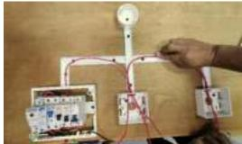
Insert one live cable from the second terminal box through the casing to the round
