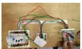
Fit the live cable (red cable) at the same 32A miniature circuit breaker and fit the neutral cable (black cable) and ground cable (green cable) at each terminal in the distribution board (DB).
