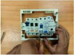
• From the lower side of residual current circuit breaker, connect it with the live cable to the miniature circuit breaker.
