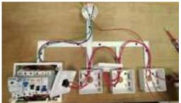
• Fit the live cables at the third terminal box to the second two-way switch. The live cable from the round PVC block is screw to the terminal common (C) and the two live cables from the intermediate switch are screw to the terminal L1 and L2
