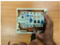
• Connect all the miniature circuit breaker together with the live cables.
