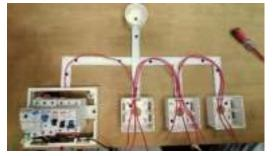
Insert one live cable from the second terminal box through the casing to the round
