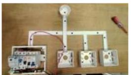
• Insert 2 live cables from the first terminal box to the second terminal box. The second terminal box will be the base for the intermediate switch.
