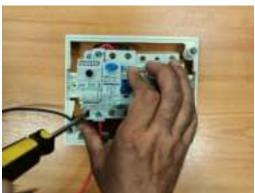
Connect the green cable to the left terminal and this will be the ground terminal. The
