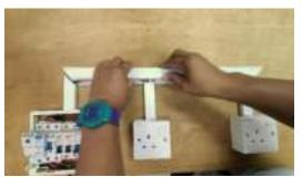
• Turn on the switch at main switch, residual current circuit and miniature circuit breaker. Finally, use the socket tester to test the functionality of the socket outlets.
