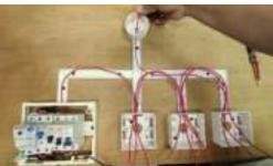
• Fit the neutral cable (black cable) at the neutral terminal. Then insert the neutral cable from the distribution box to the round PVC block.
