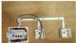
• Insert another live, neutral and ground cables from the first terminal box to the second terminal box. The second terminal box will be the base for the second socket outlet.
