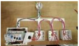
• Fit the live cables at the second terminal box to the intermediate switch. The live cables from the first two-way switch are screw to the terminal L1 and L3 and the two live cables from second two-way switch are screw to the terminal L2 and L4
