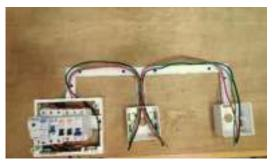
• Twist together two live cables at the first terminal box and fit it to the live terminal at the first socket outlet. Repeat the same step with the neutral and ground cables
