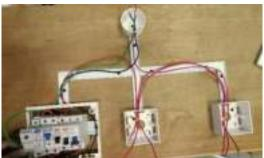
• Fit the live cables at the first terminal box to the first two-way switch. The live cable from distribution box is screw to the terminal common (C) and the two live cables from second two-way switch are screw to the terminal L1 and L2
