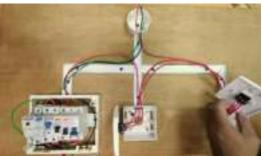
• Fit all the live, neutral and ground cables at the round PVC block to the lamp holder.
