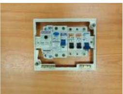
• Connect the red cable as the live cable from the upper side of the main switch to the residual current circuit breaker. The size of the cable is 16mm<sup>2</sup>.
