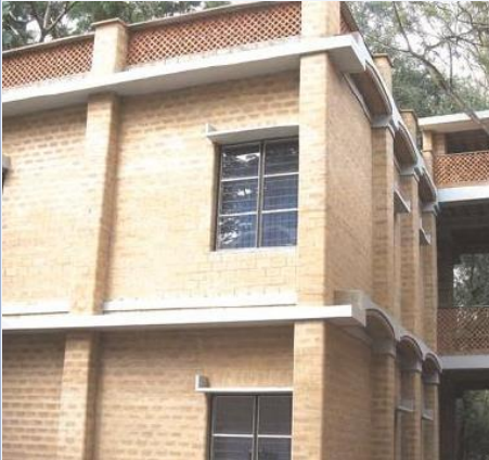
Load Bearing Walls Using Bricks Construction
