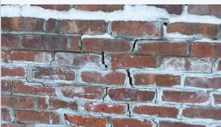
Frost Action on Bricks
