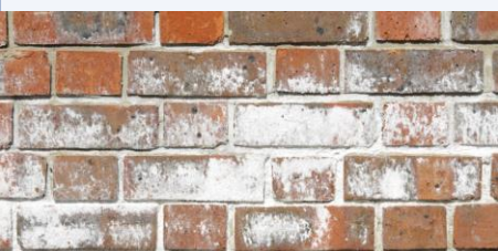
Efflorescence on Bricks
