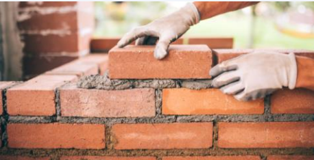
Sharp Edges and Regular Surface of Bricks
